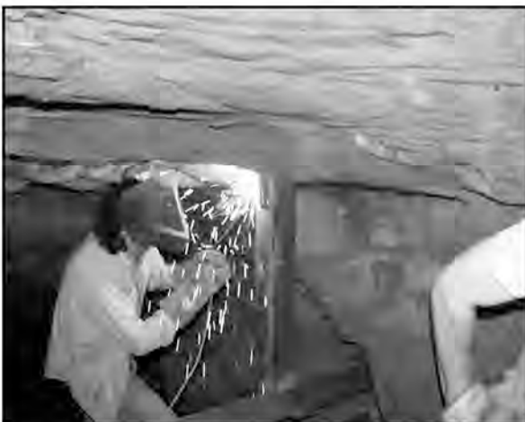
Keith Dunlap arc welding the one-inch diameter anchor pin to the vertical support on the Nyesville gate.
