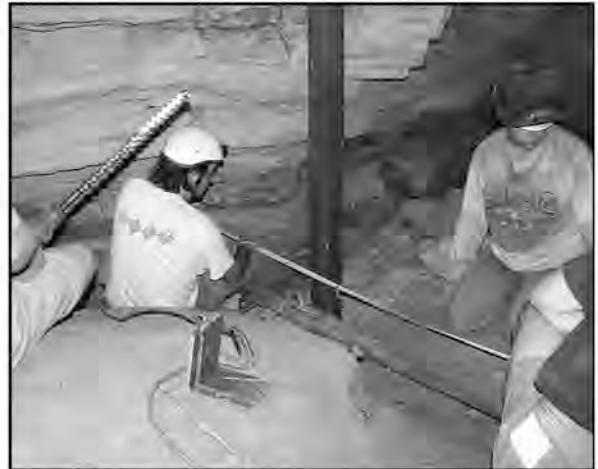
With the base-plate and vertical columns in place, it's just a matter of measuring the horizontal bar lengths and welding them in place. Note hammer-drill used to put in anchor pins.
