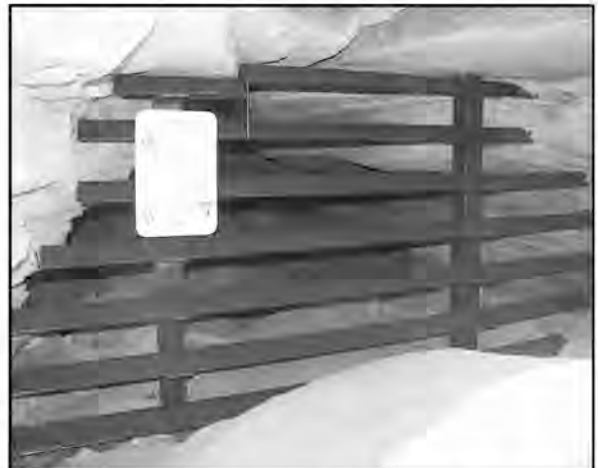
This is the finished view of the gate under construction in the above frame. The sign mounted on the gate explains that the mine is ideal habitat for bats.
