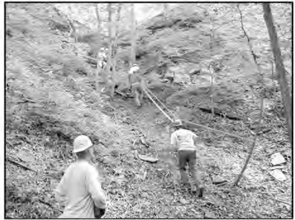
The two mine entrances at the Montezuma work site were located at the top of very steep slopes so material had to be hauled up with a tyrolean line.
