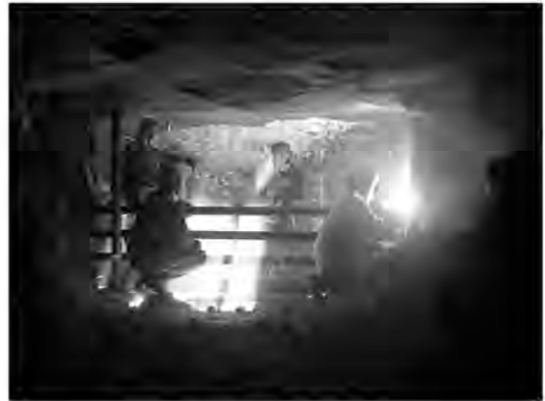
The "gate crew" working in the entrance of South Gardner mine. At the location of the gate, the tunnel was 16 foot wide by 6 foot high.
