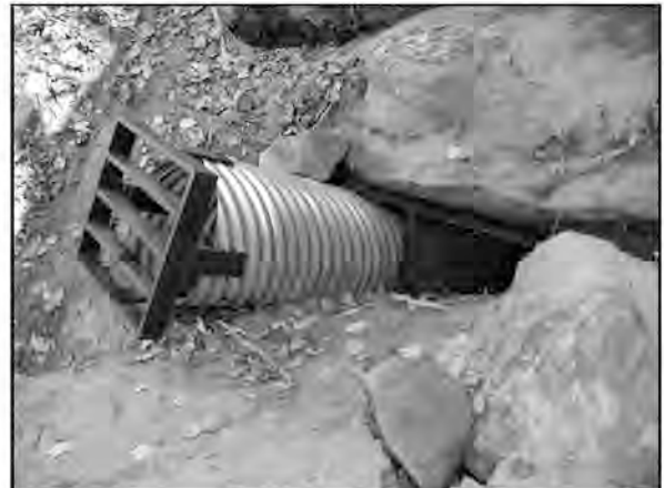
Because of their smaller size and instability, a 10-foot long by 24-inch diameter culvert was installed into this mine entrance. A pre-fabricated grate was then welded on the open end.
