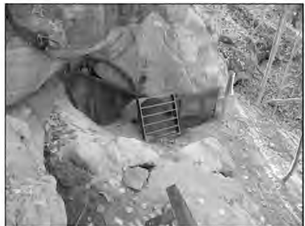
Adjacent to the entrance shown above is another entrance which used a 30-inch culvert. Framing and expanded metal mesh was then used to secure the rest of the opening.
