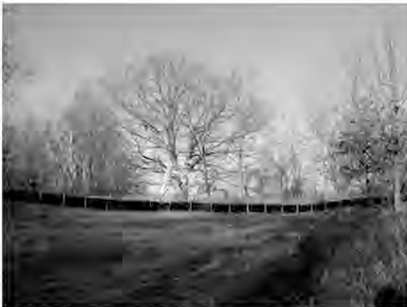
A construction silt barrier protects a sinkhole under the watchful eye of a 200 year old Oak tree.
