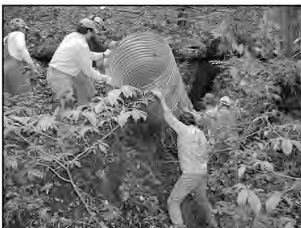
IKC volunteers inserting the 36-inch culvert into the abandoned mine entrance on the Hoosier NF.
