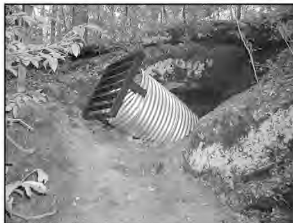
The finished culvert gate with the steel grate, restricting human entry, but allowing bats and other "cave-dwelling" biota to enter and use the mine.
