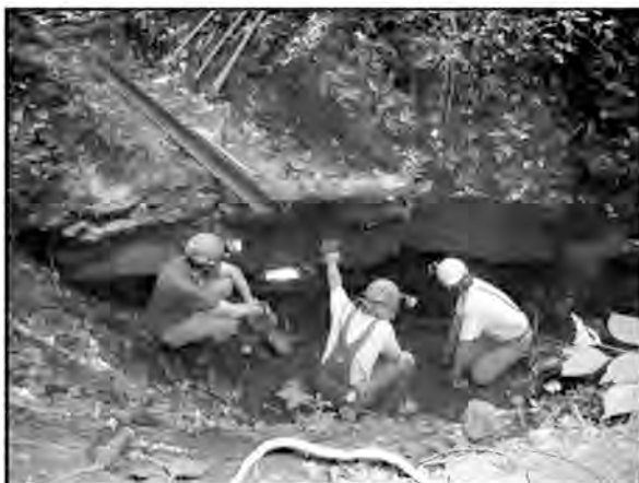
An abandoned mine entrance in Parke County having the angle-iron installed. photos by Bob Vandeventer
