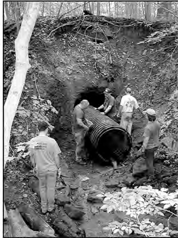
The "culvert crew" with the 36-inch diameter plastic culvert partially inserted into the second mine entrance at the Parke County work site.
