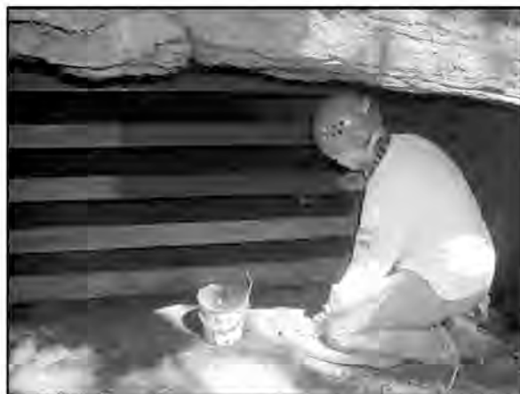
After an angle-iron gate is constructed, it must be cleaned with mineral spirits, primed, and then painted. This task generally falls upon Bambi Dunlap (in addition to her role as resident caterer).
