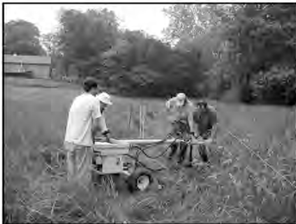
Steve Lockwood, Everett Pulliam, Mark Sparks, and Keith Dunlap operate the counter-balanced power auger to drill a 12-inch diameter post hole 48-inches deep.
