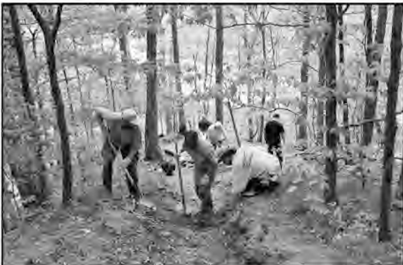
Take Pride in America volunteers working to install water bars on the trail below Patton Cave.
