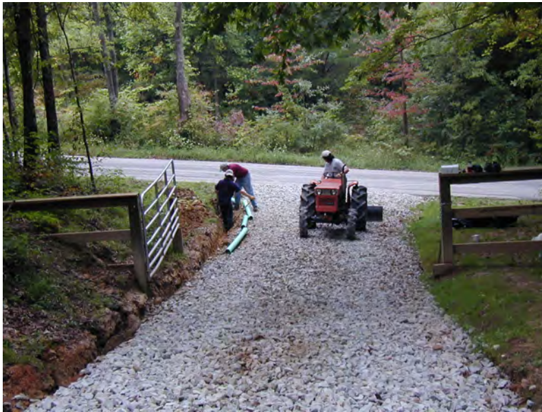
Grading the stone and installing the drainage tile along the edge of the driveway.
