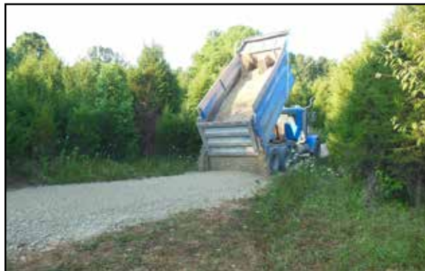
Above left: three “before” photos of the driveway. Above right: the same three locations after grading and stoning. Below left: Jamie Winner grading ruts and preparing side drainage. Below right: Tri-axle truck spreading crushed stone.
