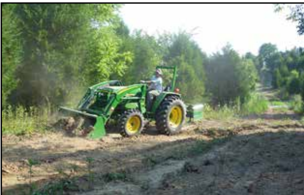
Above left: three “before” photos of the driveway. Above right: the same three locations after grading and stoning. Below left: Jamie Winner grading ruts and preparing side drainage. Below right: Tri-axle truck spreading crushed stone.
