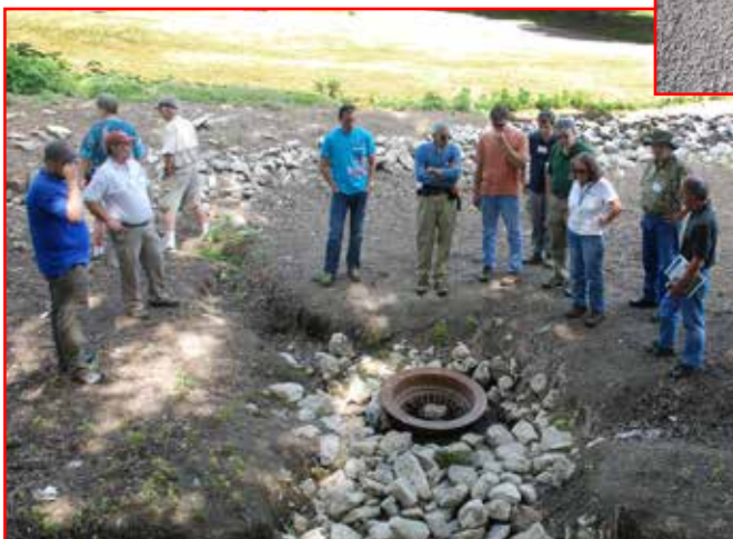
Above: InDOT’s way of “dealing with” a sinkhole containing a cave discovered during the widening of SR37. They will use over 500 tons of crushed stone to stabilize this karst feature by the time they are done (at least for the time being).
