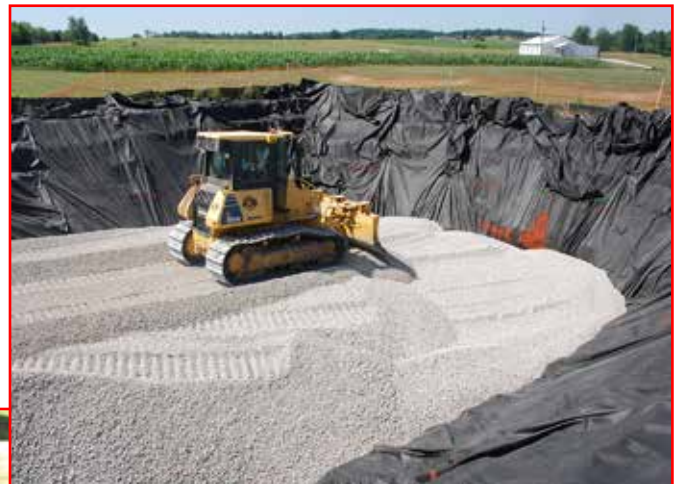
Above: InDOT’s way of “dealing with” a sinkhole containing a cave discovered during the widening of SR37. They will use over 500 tons of crushed stone to stabilize this karst feature by the time they are done (at least for the time being).
