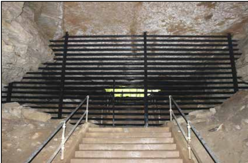
The finished Wyandotte Cave gate constructed by the IKC in July.
