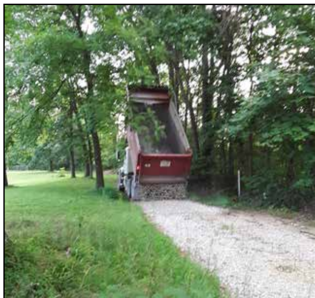
Spreading crushed stone on the old county road at Lowry.
