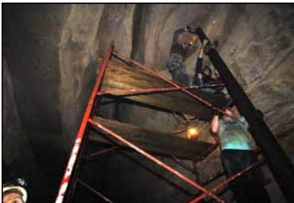
below the first horizontal bar into the water. We used a "scribing" technique to measure and cut each bar to the proper length to exactly match the contour of the floor. This worked perfectly, but took more time than I anticipated.
