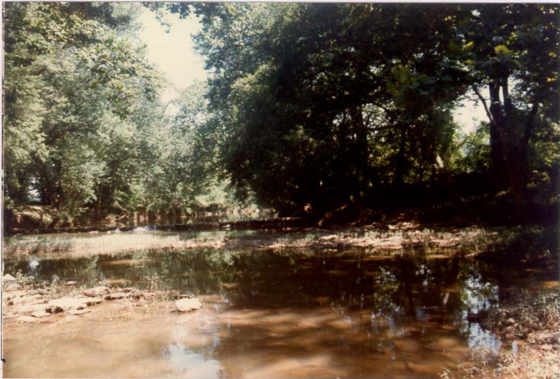
A view of the dam constructed across Indian Creek taken approximately 150 downstream below the dam (photo point 3).
