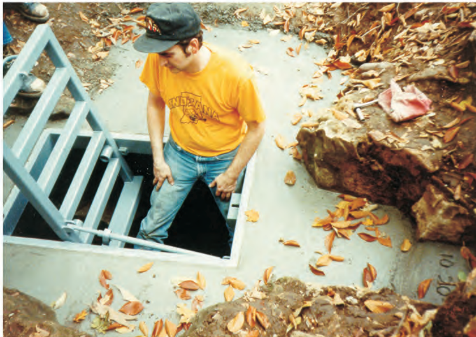
The gate with the door in the open position. Note the safety latch that locks the door in the open position and allows the door to be used as one climbs out the entrance.
