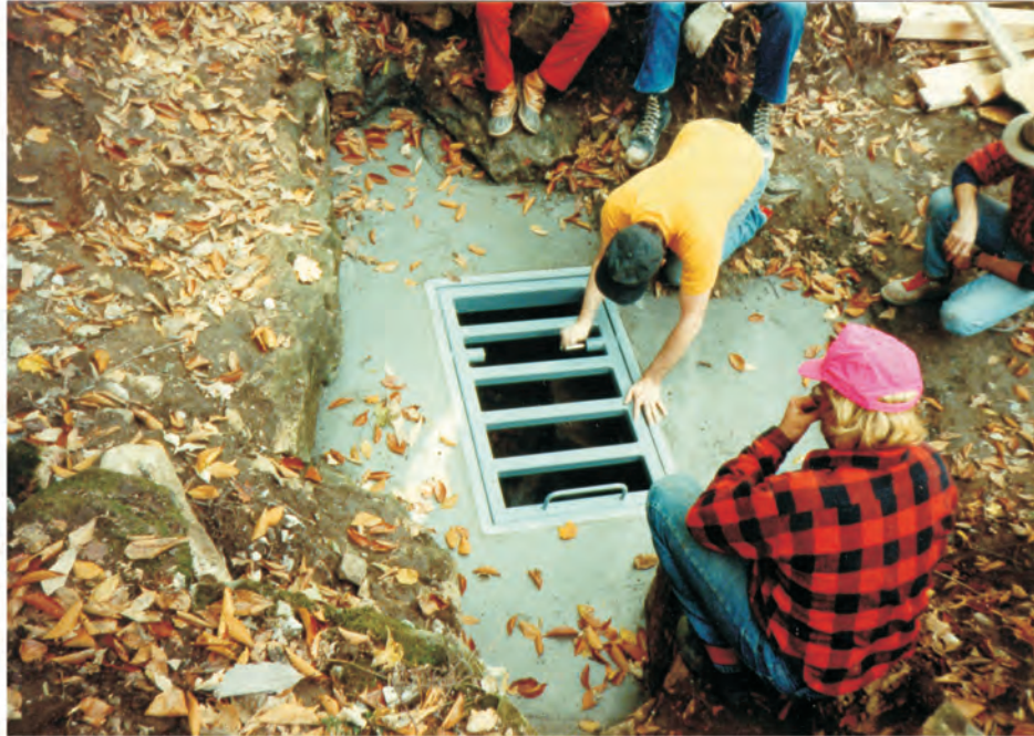
The new gate in place. The gate door measures 24" by 40" for ample air and water flow. A considerable amount of dirt and rocks had to be removed around the entrance for provide a solid foundation for the gate and concrete.
