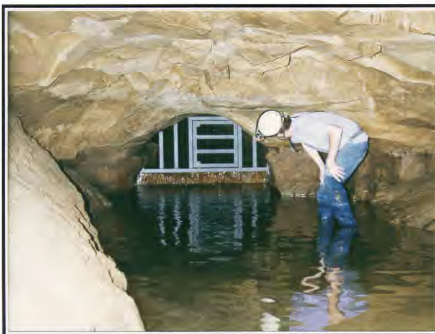
Quarry entrance gate installed in August, 1994. Inner dam visible below gate. Passage can flood to ceiling during high flow conditions.
