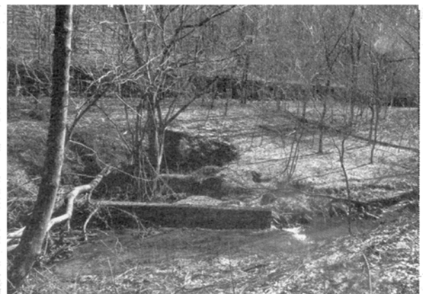
The March, 1943 swallowhole, now the entrance to Jenny Lind Run Cave. The dam was built at the cave's entrance to divert the water downstream. Behind the cave entrance is the Jenny Lind Flume. A remnant of the railroad trestle undermined by the acid is barely visible to the far right.
