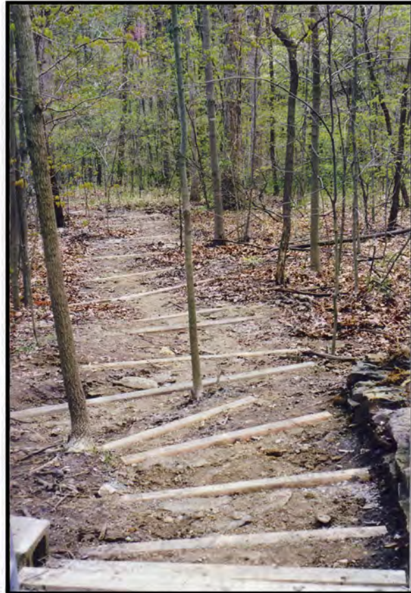
Trail from SR 54 before (upper left, looking north towards the road) and after (upper right, looking south down hill) water bars were installed. Bruce Trotter and Ray Sheldon (below) cutting re-bar used to anchor the water bars in place.
