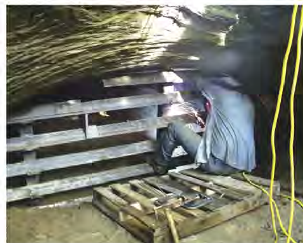
Keith Dunlap welding on the nearly complete gate #1.
