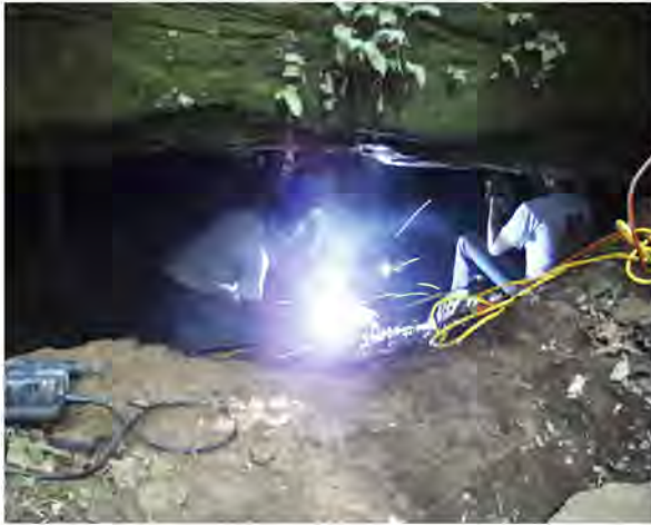
Richard Newton arc welding on gate in entrance #1.
