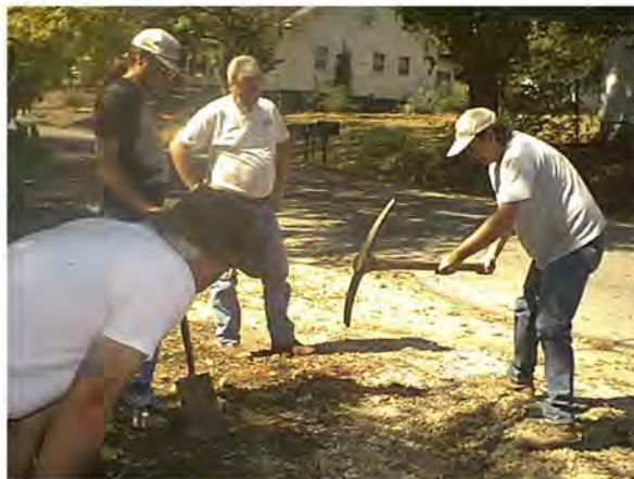
Several IKC members excavating for an old survey corner pipe defining the Orangeville Rise property boundary. The pipe was not found.
