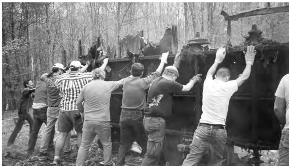
Demolition of the abandoned travel trailer.
