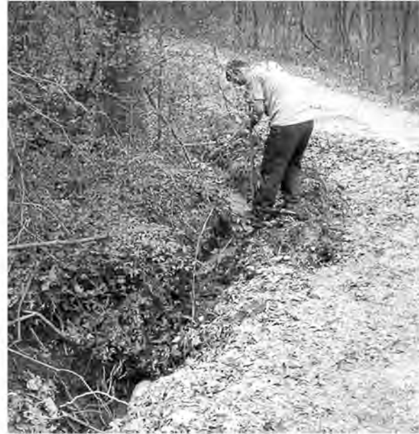
Jamie Winner digging on the access lane ditch to improve drainage.
