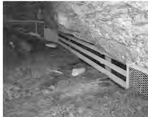
A partial panoramic view of the 98-foot wide semi-circular gate constructed in the sandstone shelter. Two 16-foot sections (left and right ends) used horizontal angle-iron construction to allow bat use. The remaining entrance openings were secured with framed expanded metal mesh pinned to the walls.
