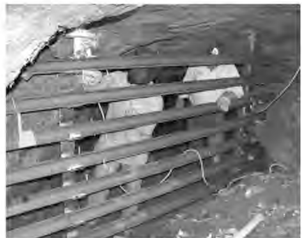
Bob Zatarski (welding) and Gene Pelter finish the construction of the mine gate located near Rockville.
