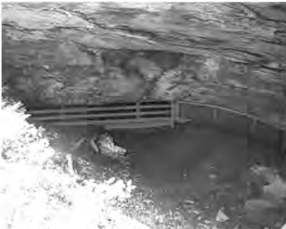
A partial panoramic view of the 98-foot wide semi-circular gate constructed in the sandstone shelter. Two 16-foot sections (left and right ends) used horizontal angle-iron construction to allow bat use. The remaining entrance openings were secured with framed expanded metal mesh pinned to the walls.
