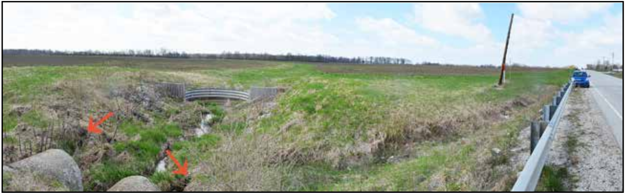
Systems of drainage lines are commonly placed under farm fields in Indiana to make them dry enough to cultivate. The groundwater is piped to the edges of the fields where it is drained into ditches or creeks. These drain tile outlets frequently are excellent places to find groundwater crustaceans that have accidentally been washed out of the soil. Shown here is the location of two drain tile outlets (indicated by arrows) in Vigo County, Indiana where a new species of isopod has been discovered.
