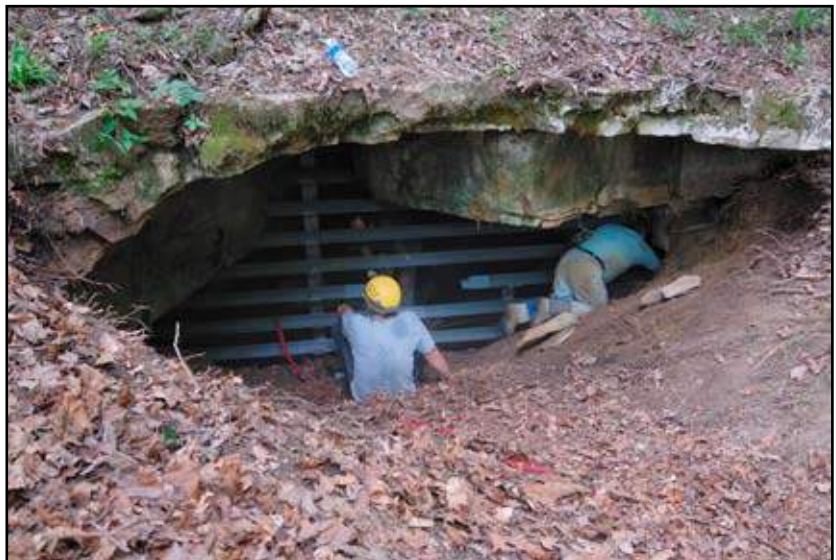
Jim Kennedy (sitting) and Ray Sheldon (right) in front of the nearly completed bat-friendly gate in the entrance to Bat Cave.
