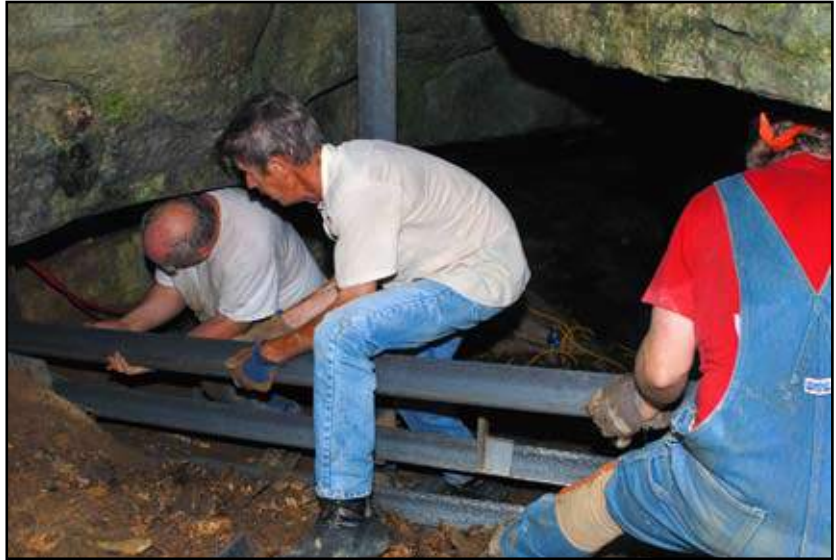
Tom Sollman, Bob Sergesketter, and Bruce Trotter positioning the third angle-iron horizontal bar in the entrance of Bat Cave.
